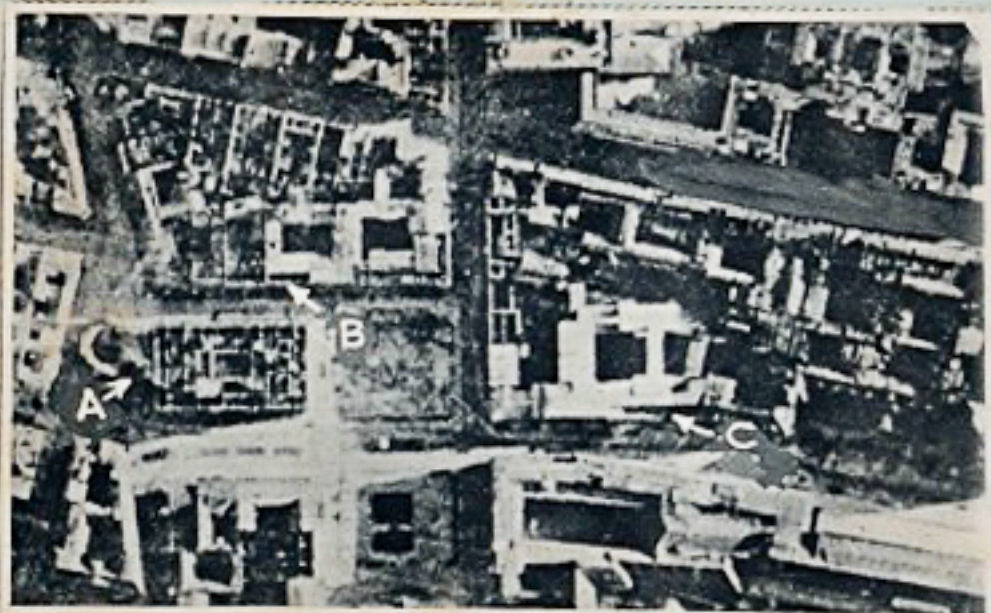
MORE DAMAGE IN THE CENTRE OF THE CAPITAL: (A) TOP FLOORS OF KAISERHOF HOTEL BURNED OUT; (B) TREASURY ROOF DAMAGED; (C) MINISTRY OF TRANSPORT AND STATE RAILWAYS DIRECTORATE
